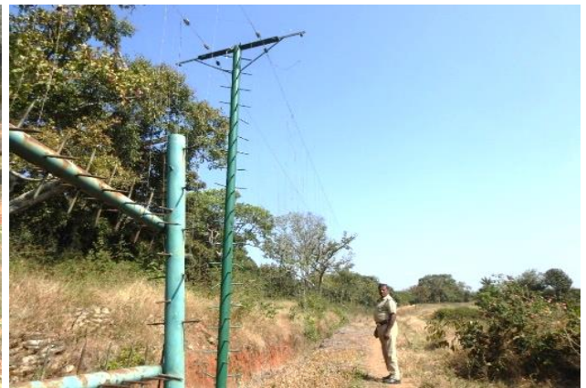
A combination of hanging and spike fence in a high human-elephant conflict zone at Hosur forest division (Photo: Milda David)
