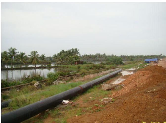
New road and pipelines (at NE1)
