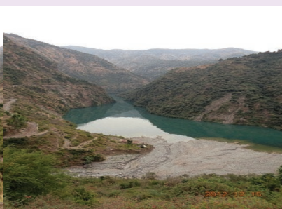
View of siltation in Ichadi Dam reservoir
