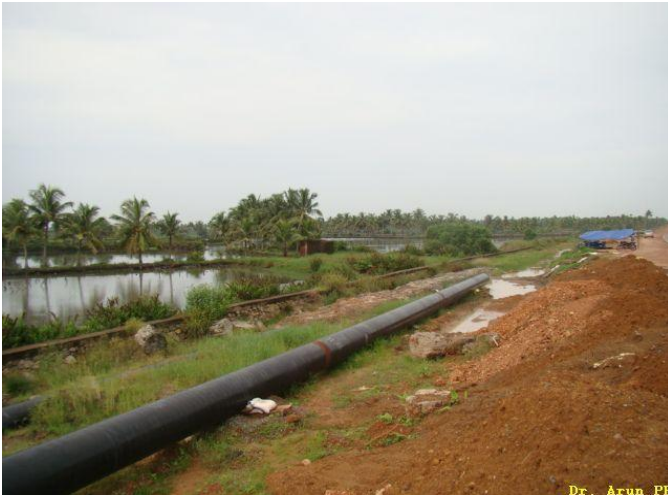
New road and pipelines (at NE1)
